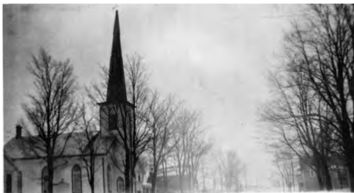
Flinton United Church before the renovation in 1962. From the 1976 commemorative booklet.
