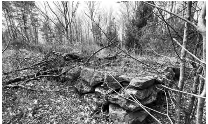
One of several foundations found along the line between Lots 41 and 42 on the Addington Road.
