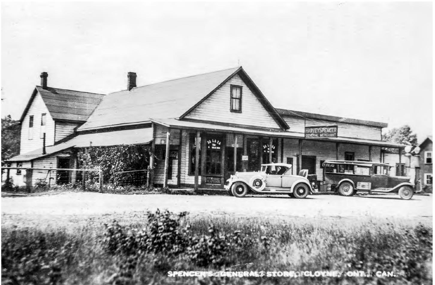
The sign on the general store in Cloyne says Harvey Spencer General Merchant. Harvey and Rachael Spencer bought the store from Rachael's father Stanley Wheeler in 1933 and ran it until 1949. You will notice that today Highway 41 is at a lower elevation than the road was when this picture was taken. Photo: Sandi Wickware Album and the Postcard Album, Flickr.
