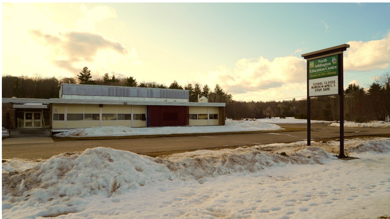
Figure 1: North Addington Education Centre Closed March 14 – April 5 – Cloyne, April 8, 2020
