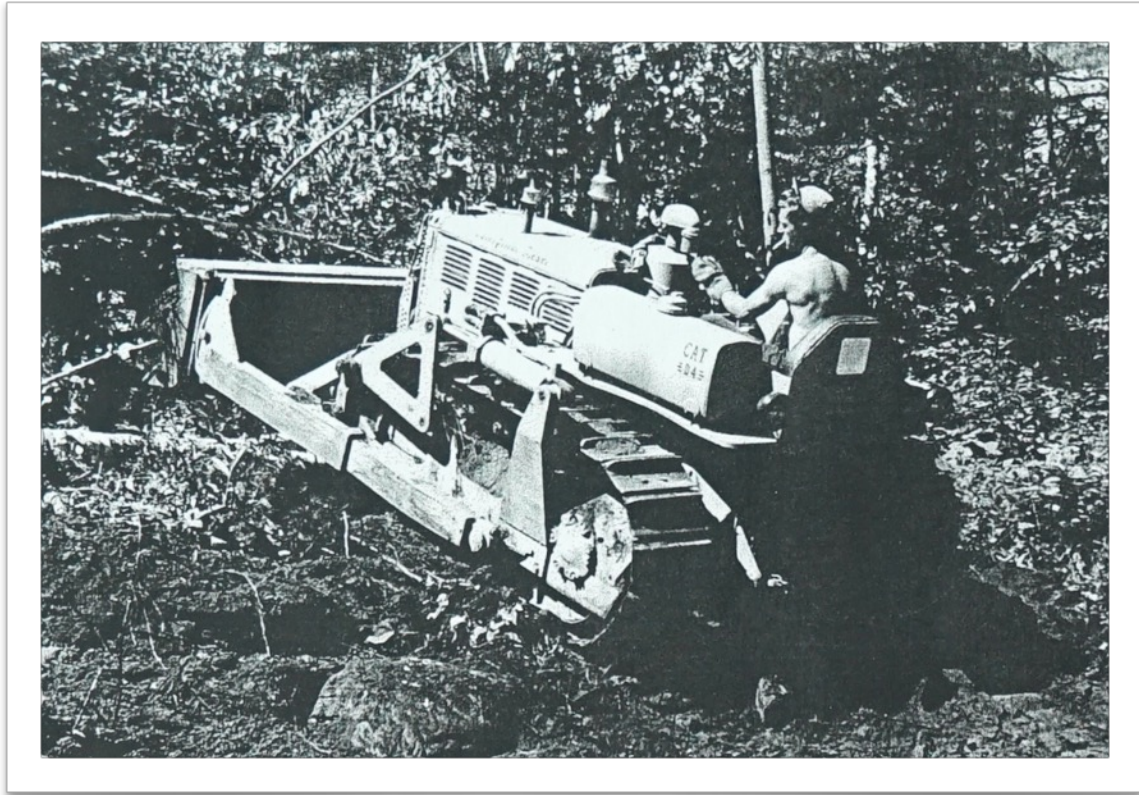
Merrill Machan Bulldozing Road at Lodge in 1950
