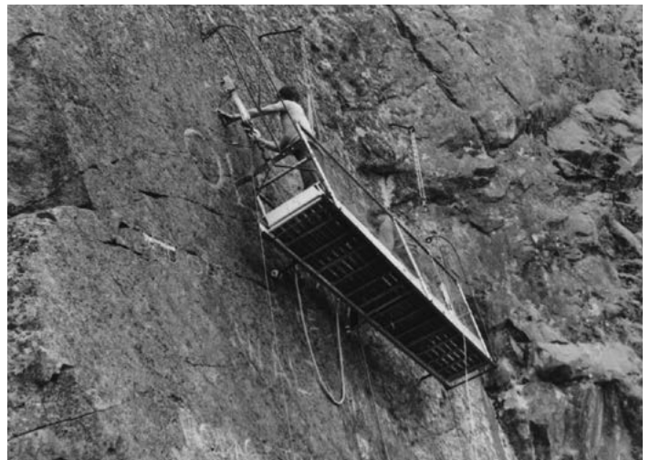
Cleaning lichen off OLD WALT, 1981. Photo: CDHS Bon Echo collection
